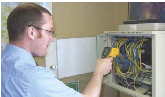
Left: Cameron undertaking an NDT infra-red check of an electrical system.
